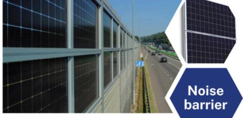
A solar noise barrier is a dual-purpose structure that combines sound insulation with solar energy generation. It typically consists of noise-reducing panels integrated photovoltaic (PV) modules, installed along highways, railways, or industrial zones. These barriers serve the dual function of reducing noise pollution and generating renewable electricity.
