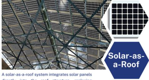
directly into the roof structure, replacing traditional roofing materials with clean energy solutions. With our proprietary leak-proof mounting structure, enjoy dual benefit of roof and solar in one solution.
