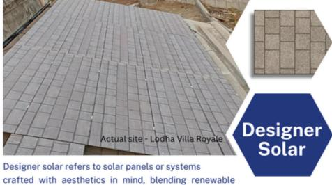
energy technology with stylish design elements. These systems, which can include customized colors, textures. or patterns, allow architects and homeowners to incorporate solar power seamlessly into a building's appearance.
